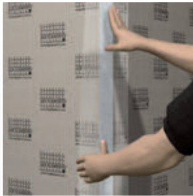
Slightly broader, self-adhesive reinforcement strips ARM-150 SK or ARM-250 SK are used for the reinforcement of corners and then levelled out with fixing adhesive COL-AK.
