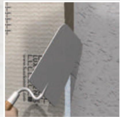
To bond the edges, e.g. for joints, apply the fixing adhesive COL-AK with a bricklayer's trowel.
