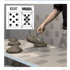
**Dots of adhesive** — Depending on the evenness of the subsurface, apply the fixing adhesive COL-AK pointwise on one side using dots of adhesive (8 — 10 dots per m<sup>2</sup>).
