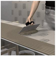
**Application with notched or smoothing trowel** — If ELEMENT-EL Baby 4 is used, **always** apply the fixing adhesive COL-AK over the full surface using a notched trowel.
